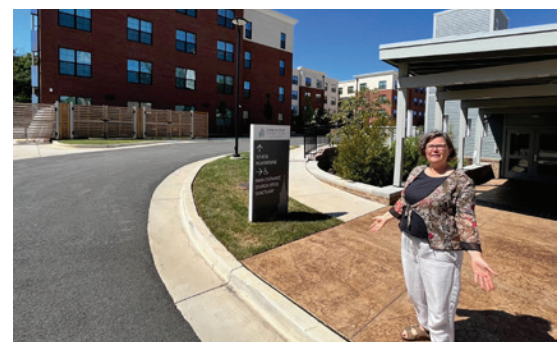
The Rev. Julie Wilson Black and Fairlington Presbyterian Church in Alexandria, Va., in National Capital Presbytery partnered with Wesley Housing Development Corporation to build The Waypoint on the FPC property that provides 81 units of affordable housing.
